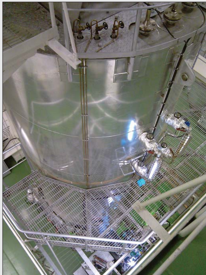
Marine Auxiliary Boiler
