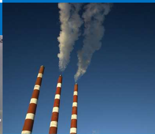
Continuous Emission Monitoring System (CEMs)
