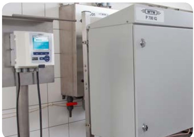
System 282/284 with Phosphate analyzer P 700 IQ
