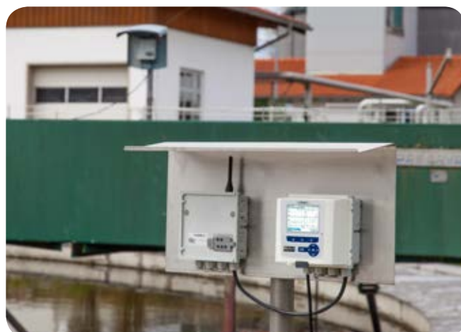
Optimal sludge level measurement with system 282/284 and radio connection
