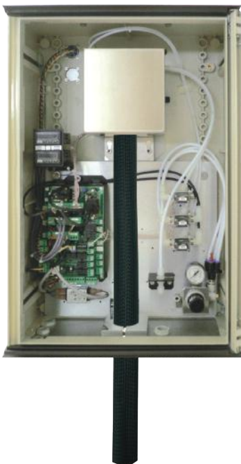
HOFI internal view with heated line correction
