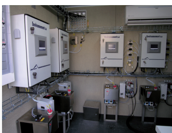
MIR 9000 - customized installation
