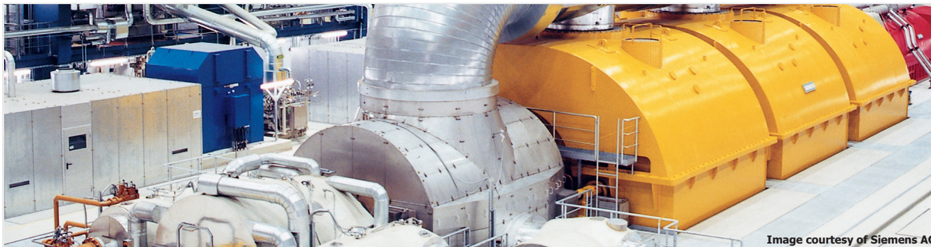
Image courtesy of Siemens AG
